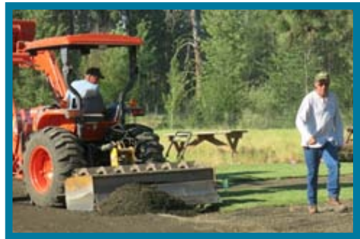
Master Hunters laying the gravel. (S.Rancourt)
