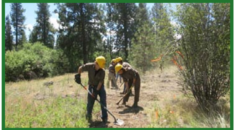
Northwest Youth Corps restoring the West Blackhorse Trail. (S. Rancourt)
