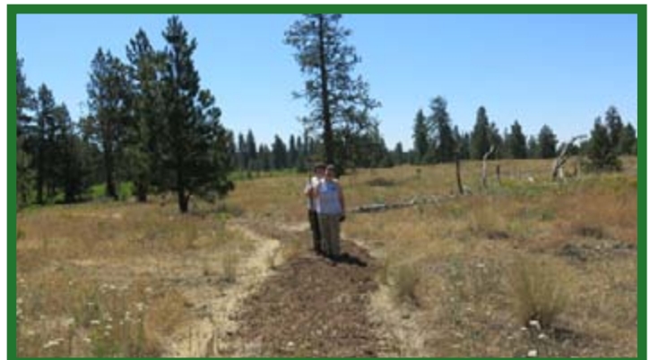
Two YCC crew members putting the finishing touches on the East Blackhorse Trail. (S. Rancourt)
